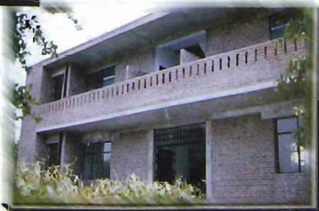
● Newly constructed Transit Flats at ISI, New Delhi
