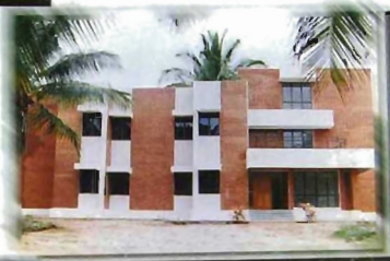
● New Hostel Block at ISI Bangalore
