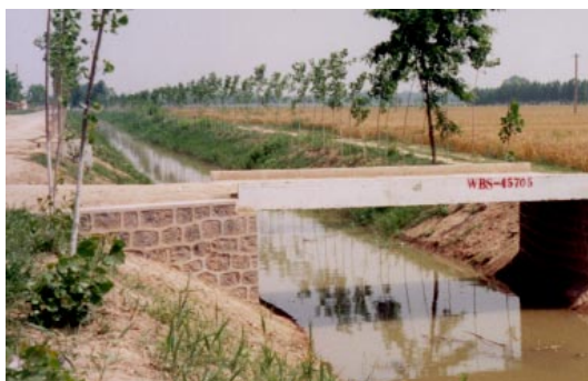
Lining irrigation canals reduces water percolation losses.
