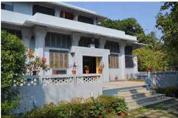
PCMM&A Building (Amrapali)
