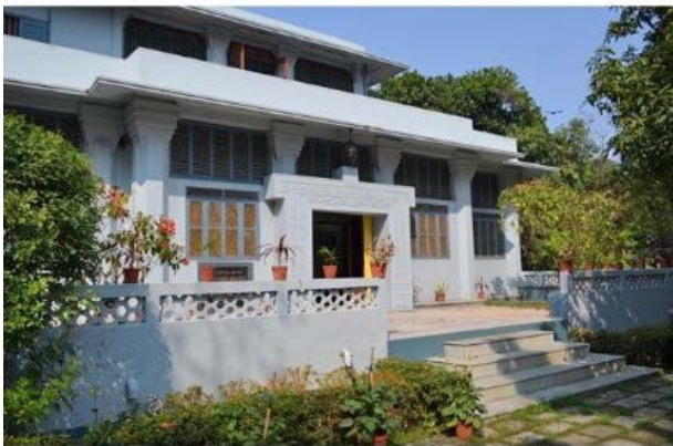
PCMM&A Building (Amrapali)
